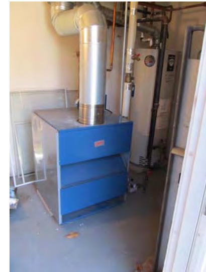
Typical central boiler and indirect-fired domestic hot water tank serving a residential building
