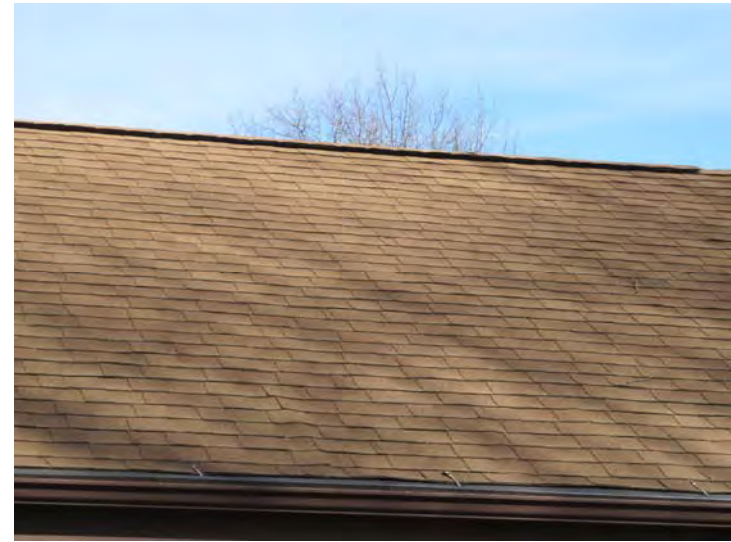
Newer architectural-style shingles that are in good overall condition are typical on all buildings
