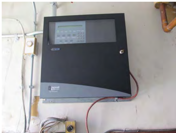
Modern, fully addressable, fire alarm control panels and new in-unit devices were recently installed throughout the development
