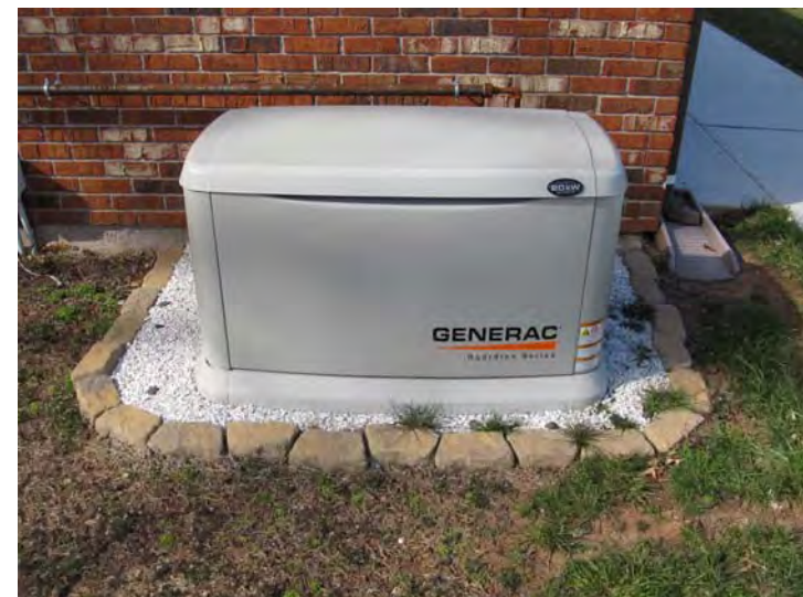
Small, recently installed, emergency generator that serves the community building
