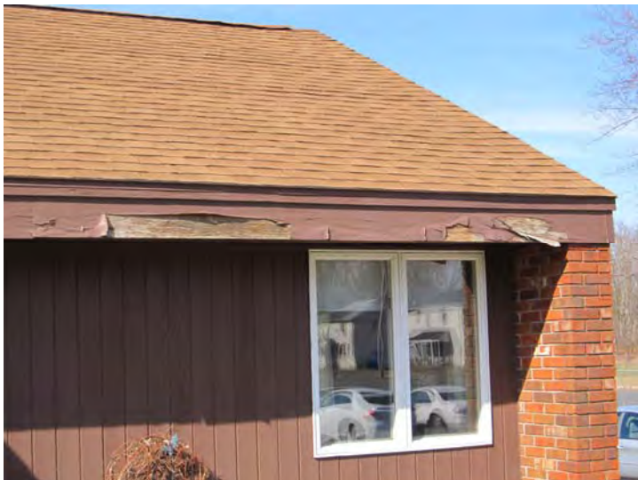
Areas of peeling paint noted on wood trim at some locations
