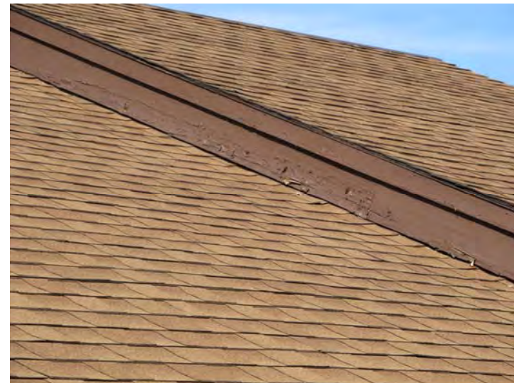
Wood rake boards at roof lines also exhibit areas of peeling paint at some locations
